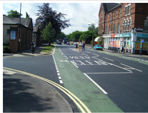
Image 6.2 Improved section of Fulford Road between Cemetery Road and Hospital Fields Road
