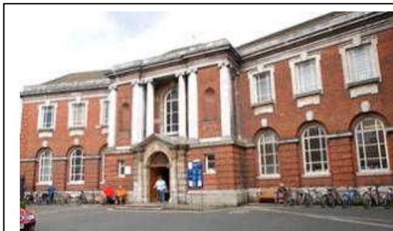
Image 5.1 Exterior of York Library
