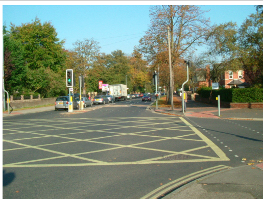
Image 6.1 Current road layout of Fulford Road between Heslington Lane and Hospital Fields Road
